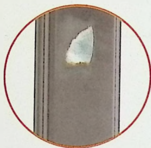
Before repair 修复前
