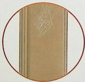
Before repair 修复前
