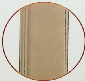
After repair 修复后
